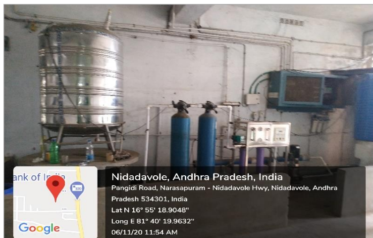
R.O. Water plant - Outlet is connected to garden
